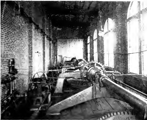
FIG. 5.—VIEW OF SHAFT HOUSE.
